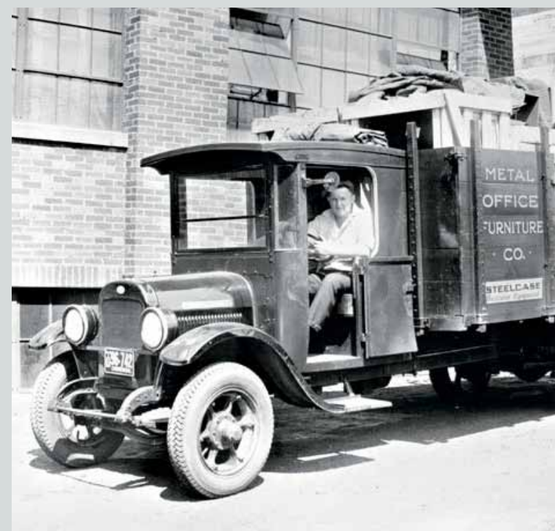
Established in 1912 as the Metal Office Furniture Company.
